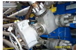
Rupture disc
